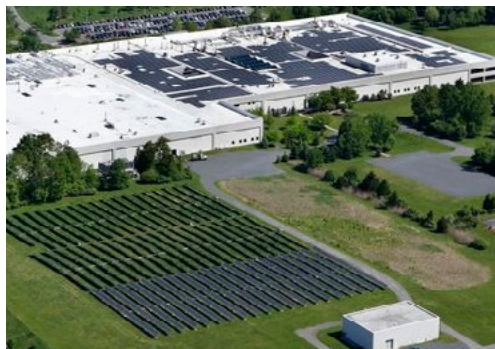
Figure 4. SunPower installation at Johnson & Johnson facility. Source Sunpower Website
