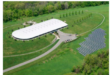
Figure 1. RGS Energy installation. Source: Real Goods ( http://realgoods.com/ ).
